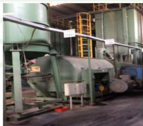
Lead Power production
